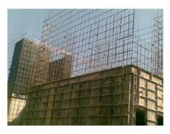
bolts at different holes, walls of 100, 150 or 200mm can be cast. Wall and Slab concrete is poured in one go for the entire floor at a time. A high-flow concrete is desirable to ensure proper consolidation. Once the concrete hardens, the bolts are removed, de-shuttering done and plates taken out of sleeves.
